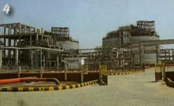
4. Project: Propane/Butane/LPG Import-Export terminal, Ennore Size: Two steel-steel double walled refrigerated storage tanks of 15,000 MT; 2 mounded Bullets - 300 MT each Value: Rs 275.79 crore Completion Date: August 2012
